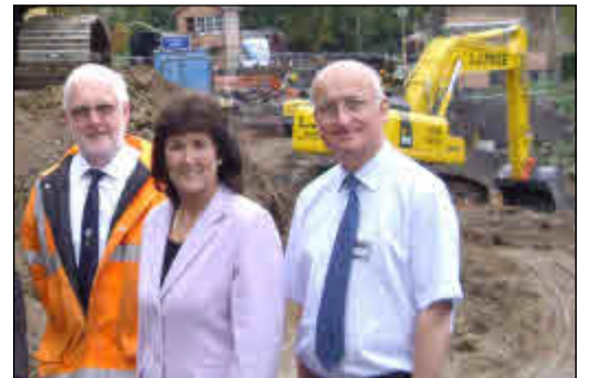
Liz at the scene of the reconstruction work on the Severn Valley Railway after the 2007 floods devastated the line.
